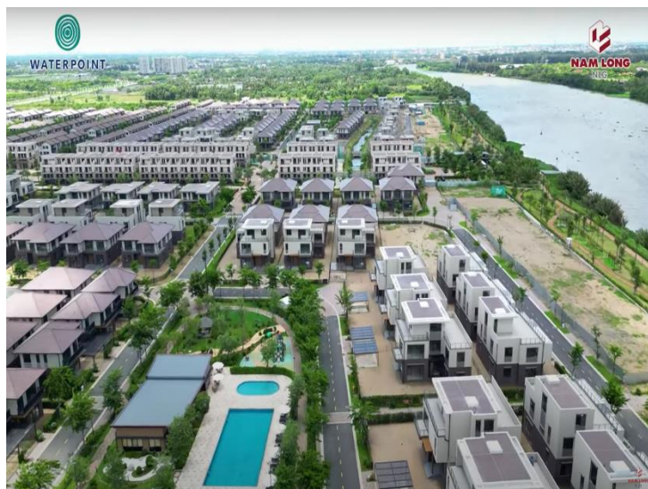
Figure 3: The Aqua subdivisions has nearly been completed
